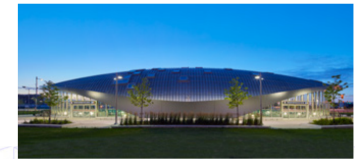
↑ Climate-responsive design The form and material of the roof is designed to support snow loads in response to the local climate.
