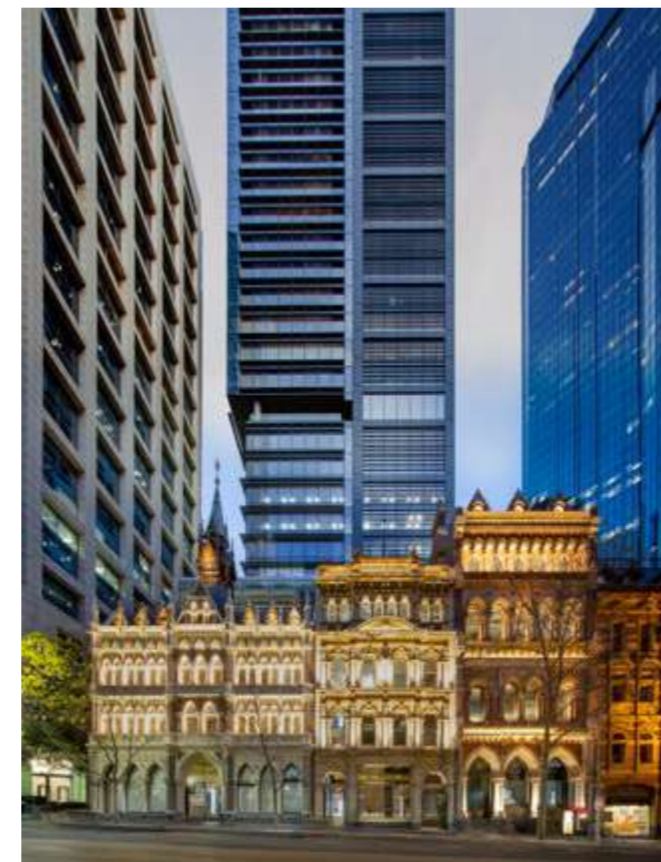
Olderfleet Buildings ↑ Integration and preservation
