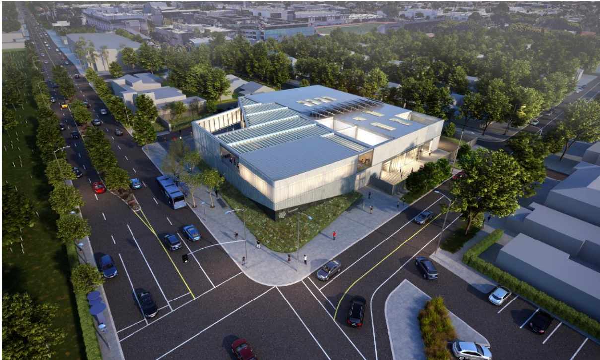
Aerial view of proposed design for the new Santa Monica College arts complex
